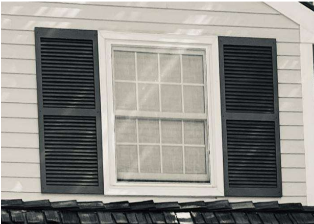
Window with correct sized shutters
