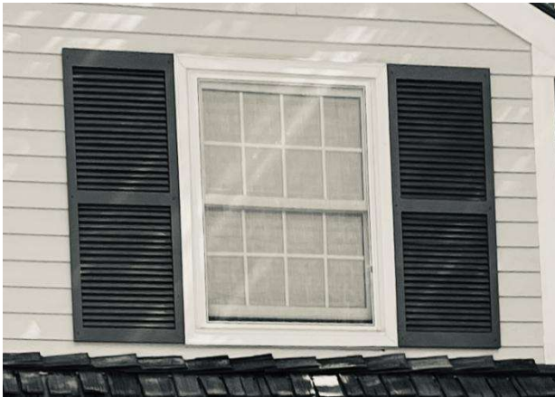
Window with correct sized shutters
